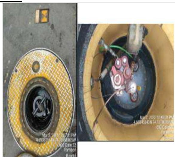
Foto 15. Bomba sumergible y Spill-container Tanque 5
