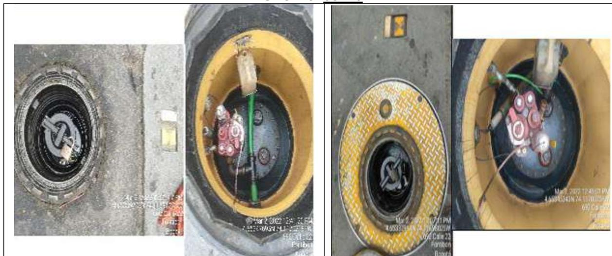
Foto 14. Bomba sumergible y Spill-container Tanque 4
